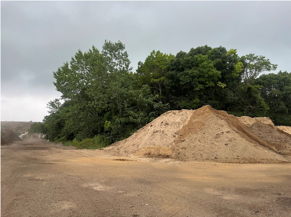
Photograph No. 6: Exterior view of woodland edge and site operations to the south of Sample Plot SP-3, facing east (July 14, 2023).
